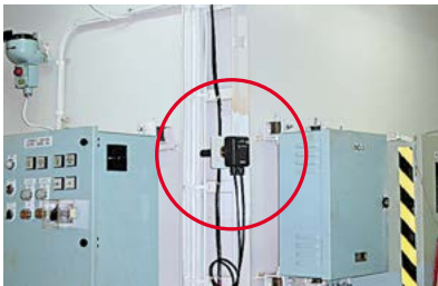
Beside rudder unit
